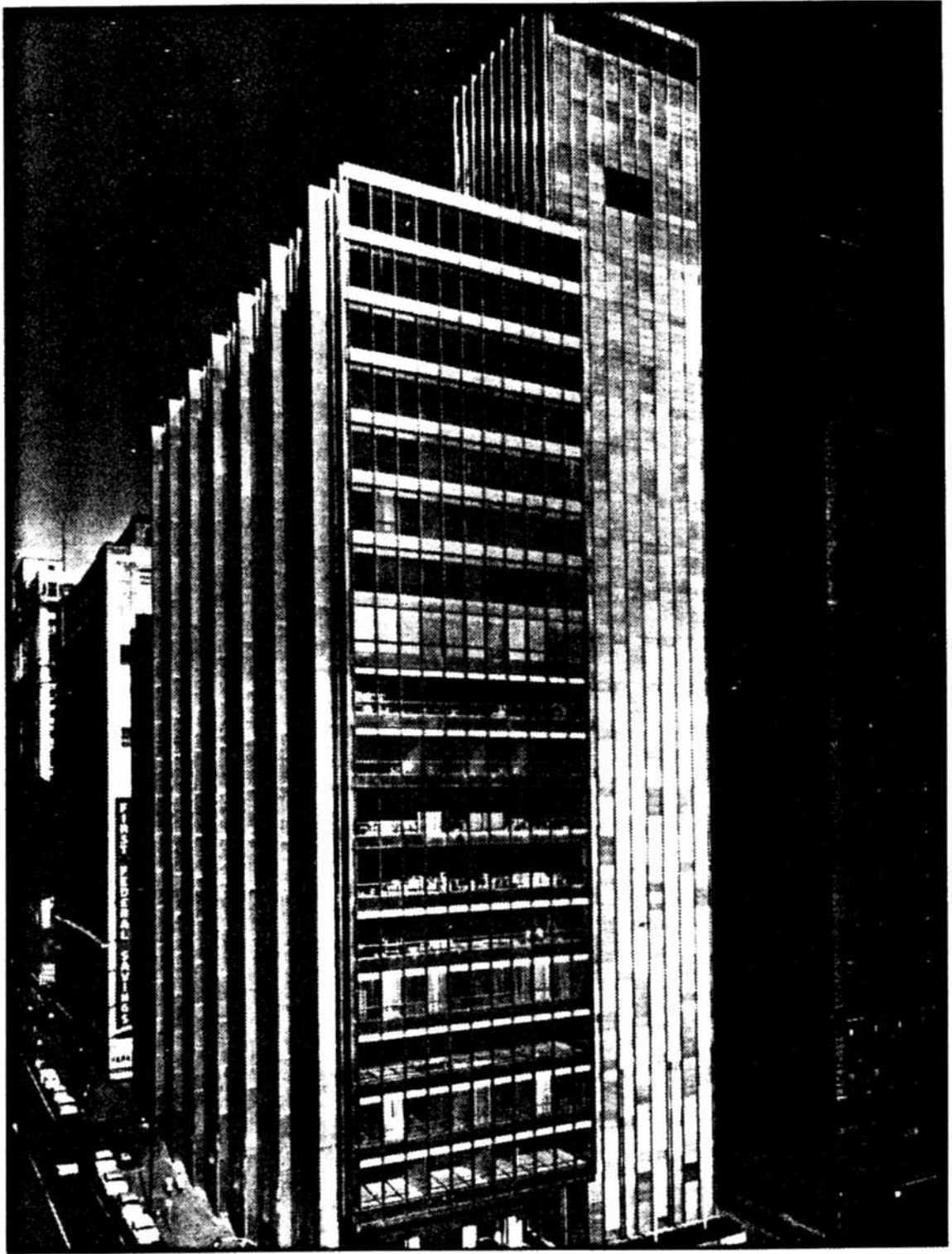
The Inland Steel Building stands in striking contrast to its neighbor, the Majestic Building (1905), which encloses its structural frame in heavily ornamented terra cotta. ( Hedrich-Blessing, photographers )
